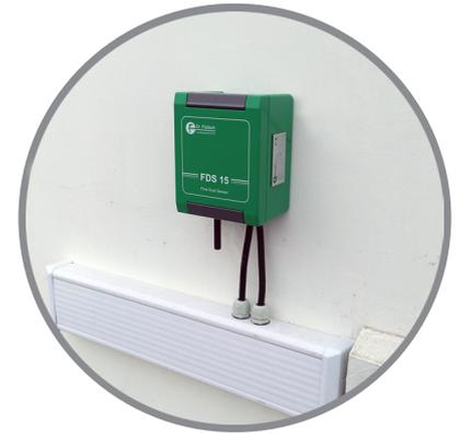
For monitoring the fine dust content at factory premises of the company SNF Floerger a FDS 15 has been mounted at the outer wall of an office building. By means of this outside installation the own production shall be controlled as well as the actual fine dust content of the ambience shall be monitored.
